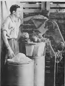
The final step is grinding of the aloin chunks into a fine yellow powder. Irving D. Cantor points to the pulverizing machine which does this. (By his right hand is a heap of the aloin powder.)
